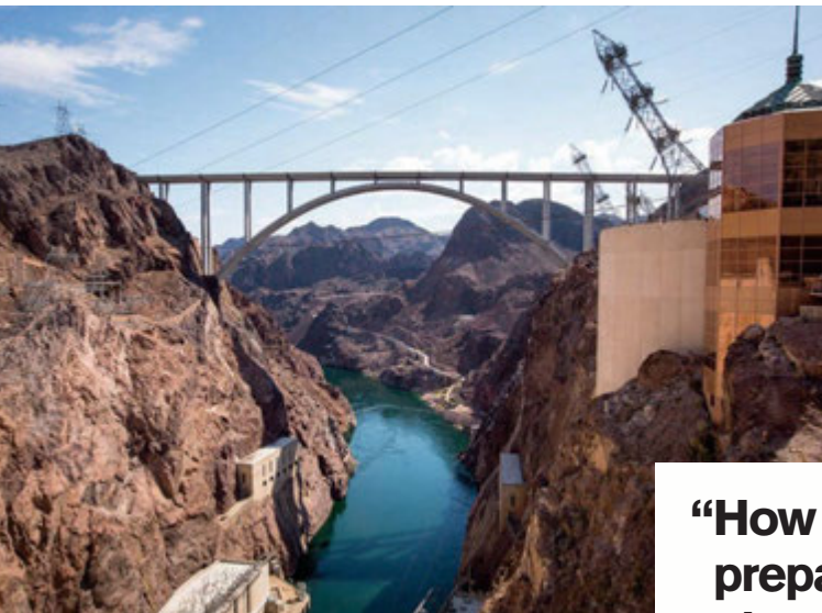
The Pat Tillman Memorial Bridge on U.S. 93 soars above the Colorado River spillway from Hoover Dam.
