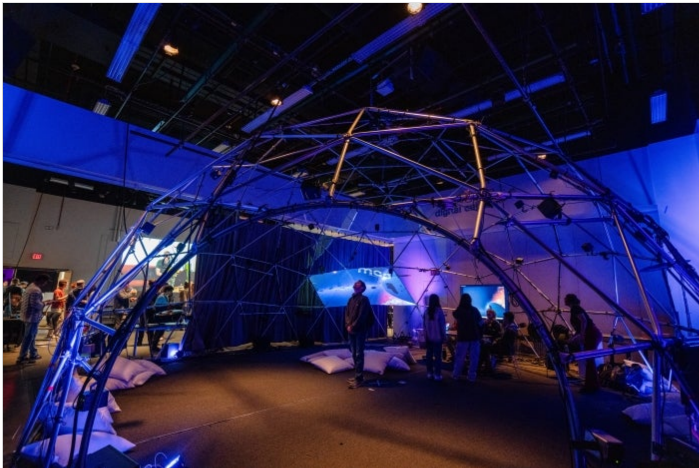
The ambisonic dome, which nearly fills room 127 in Stauffer Hall B, has 45 speakers to create an immersive sound experience. Photo by Laura Segall/ASU
