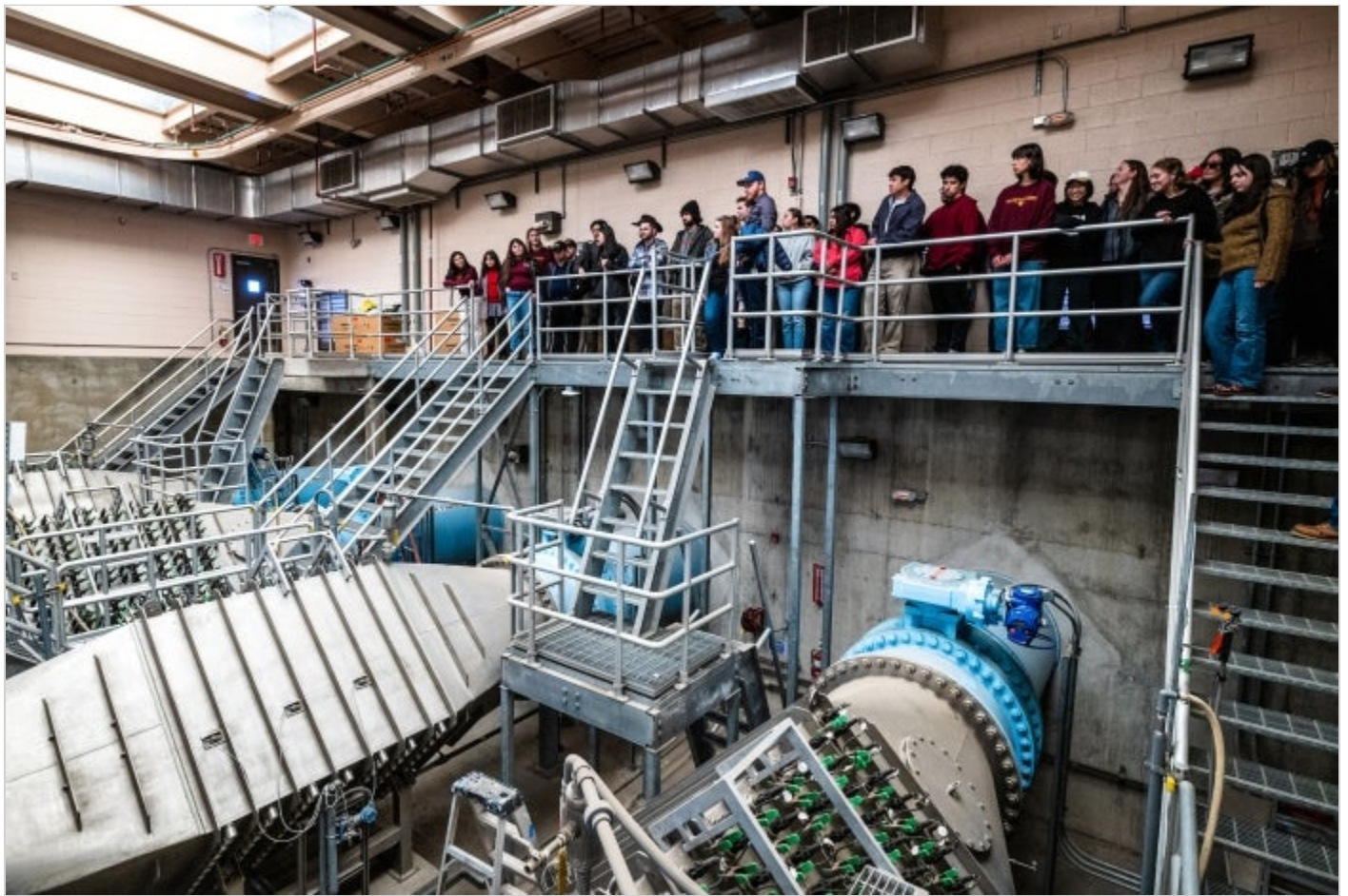
Engineering students tour the UV light filtration that deactivates bacteria and viruses from the SRP water at the South Tempe Water Treatment Plant.
